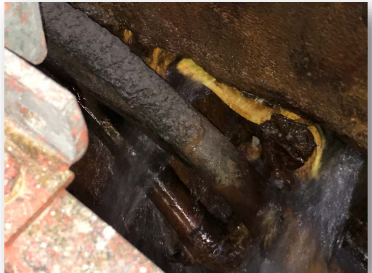
The waterproofing specialists also tested the swelling waterstop on the ingress points to ensure that the waterstop would swell to its maximum capacity to alleviate water pressure to continue with the crystalline leak repair system..
