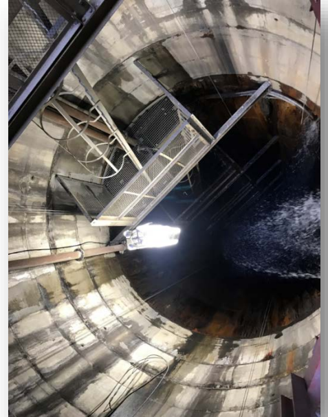
View from the top of the shaft during the site inspection. The extreme water ingress points are evident all the way down the ventilation shaft. The base of the ventilation shaft was filled with water for 35 years.
