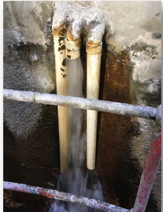
Using a rapid-setting hydraulic cement and a swelling waterstop, the waterproofing specialists were able to successfully contain the flow of water to a single access point, thus making the water more manageable.
