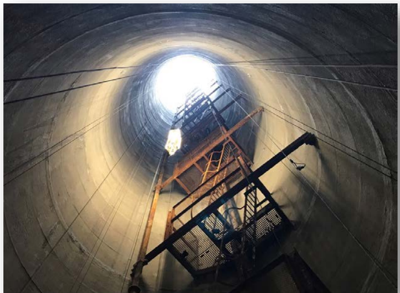
View from the bottom of the shaft once the project was complete
