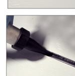
Tool away the excess joining sealant and blend the join.
