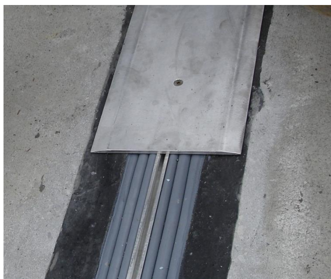
SJS SYSTEM installed with EMCRETE elastomeric nosing material in blockouts on each side of joint gap.
